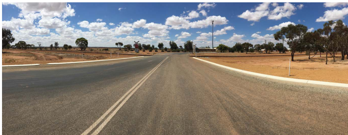
Above: North view of Railway crossing.
