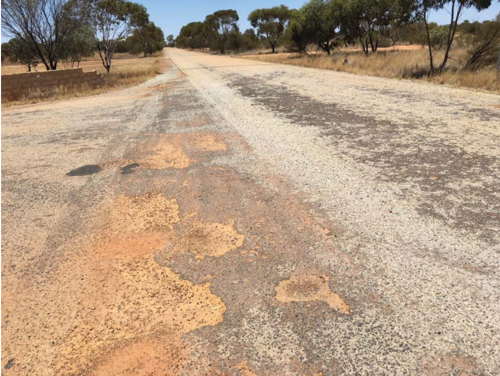
Above: Williams Drive / Earl Drive Intersection
